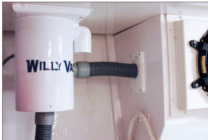
Figure 4: Vacuum Motor, Installed
